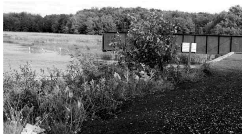
Figure 6. View east past old railway bridge towards undisturbed channel and area of weir stake concentrations (courtesy MFFC).
