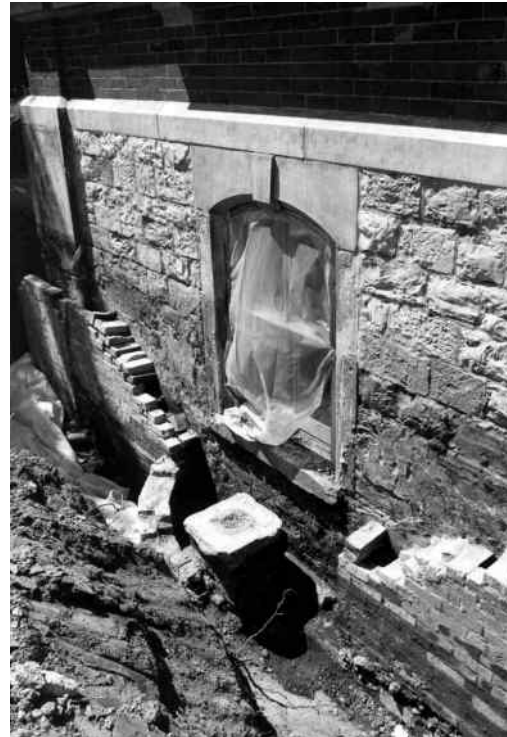
Figure 2. George Brown House, Toronto. Excavation and monitoring activities revealed a shell wall surrounding the entire foundations of the house. Photo credit Ontario Heritage Trust.
