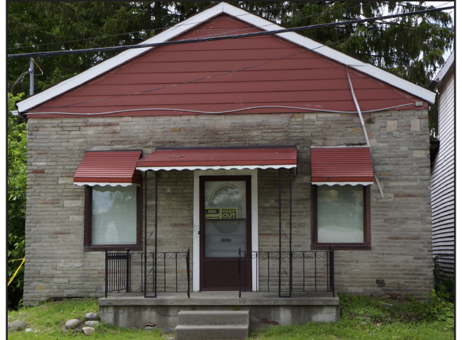
Former African Methodist Episcopal/British Methodist Episcopal Church Building, May 2013
